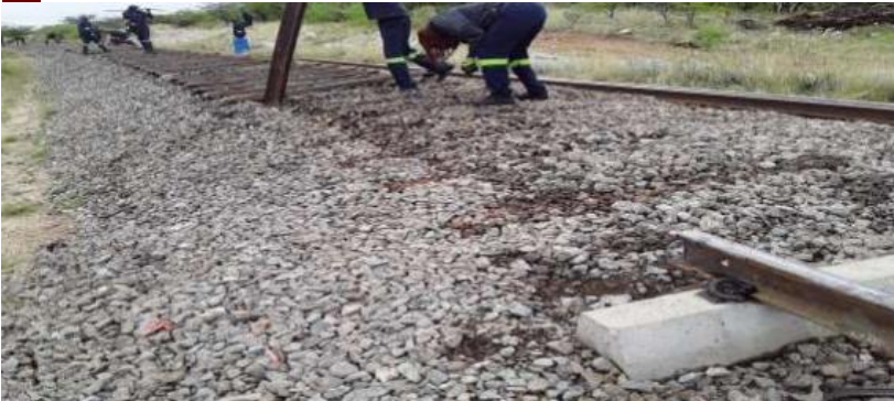
The breaking team busy removing the steel sleepers
