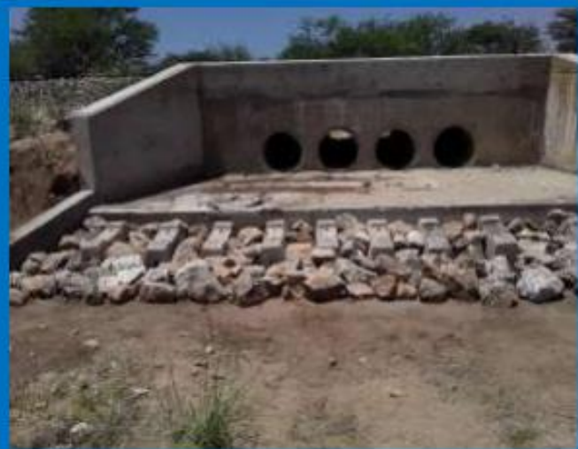
Erosion protection under construction
