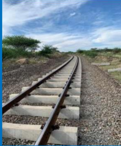
Work well done. The new railway with new concrete sleepers and no "evil" gaps that cause train derailment
