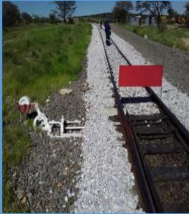
Other railway turnout/switch point. The railroad switch points help the train to be guided from one track to another. The switch points are one of the most interesting points on the railway system yet are complicated but beautiful at the same time.
