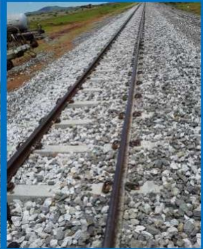
Work well done. The new railway with new concrete sleepers and no "evil" gaps that cause train derailment
