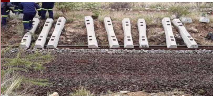
The concrete sleepers to inserted replacing the old steel sleepers
